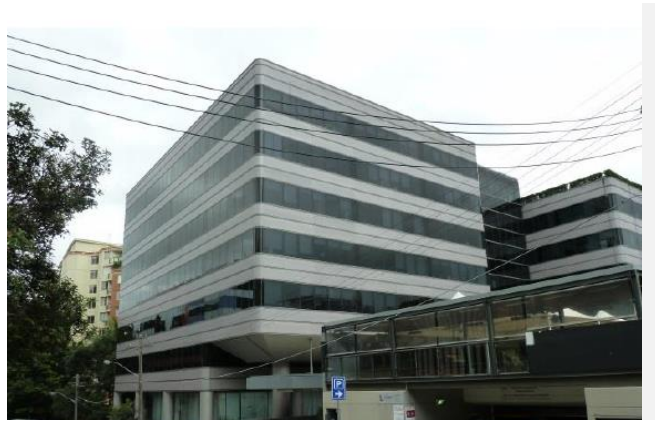
Figure 23 – Mastercard building at 72 Christie Street Source: Ethos Urban
